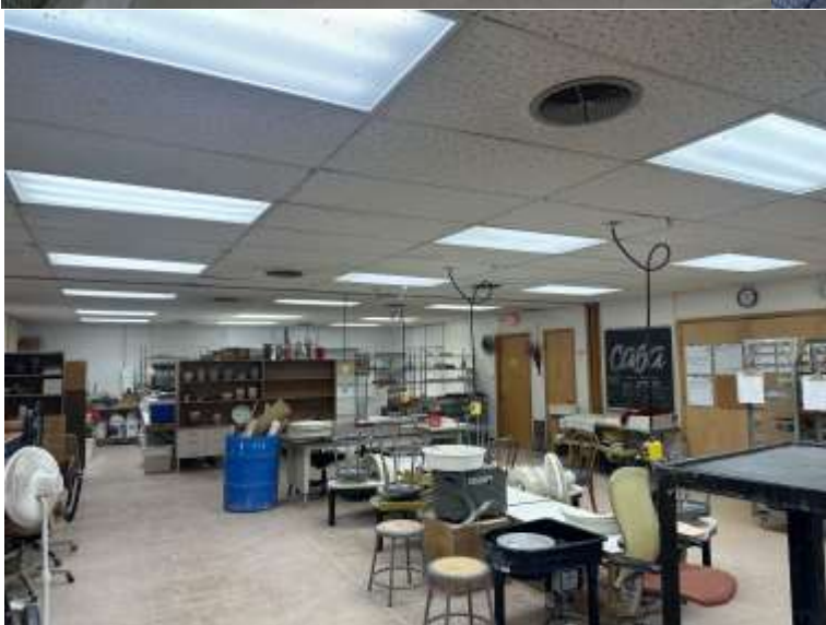
New lighting in the lower level of the Annex building
